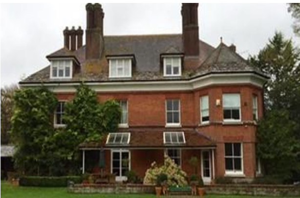
Figure 12: Baillie House on Poole Road (below)
