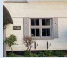
Window with external shutters
