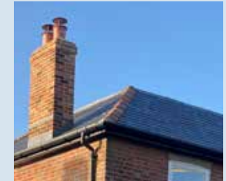
Slate roof with chimney stack built with red brick
