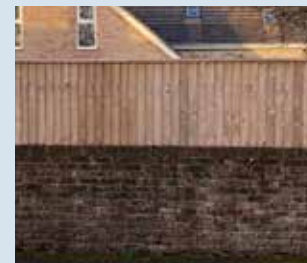
Mix of low wall with brown brick and picket fencing
