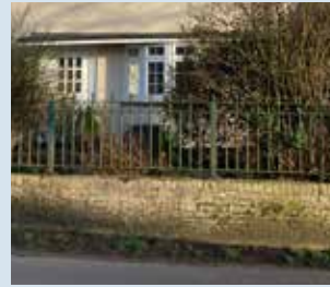
Mix of gault low bricks and railing
