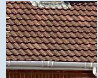
Terracotta roof ridges
