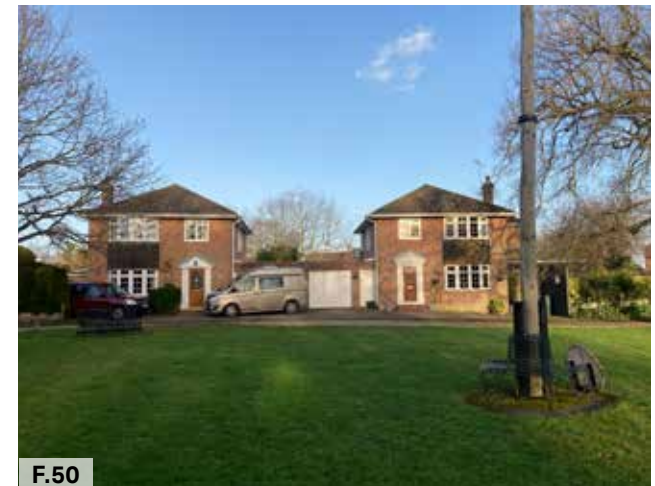
Figure 50: Detached housing looking onto a green space within the conservation area
